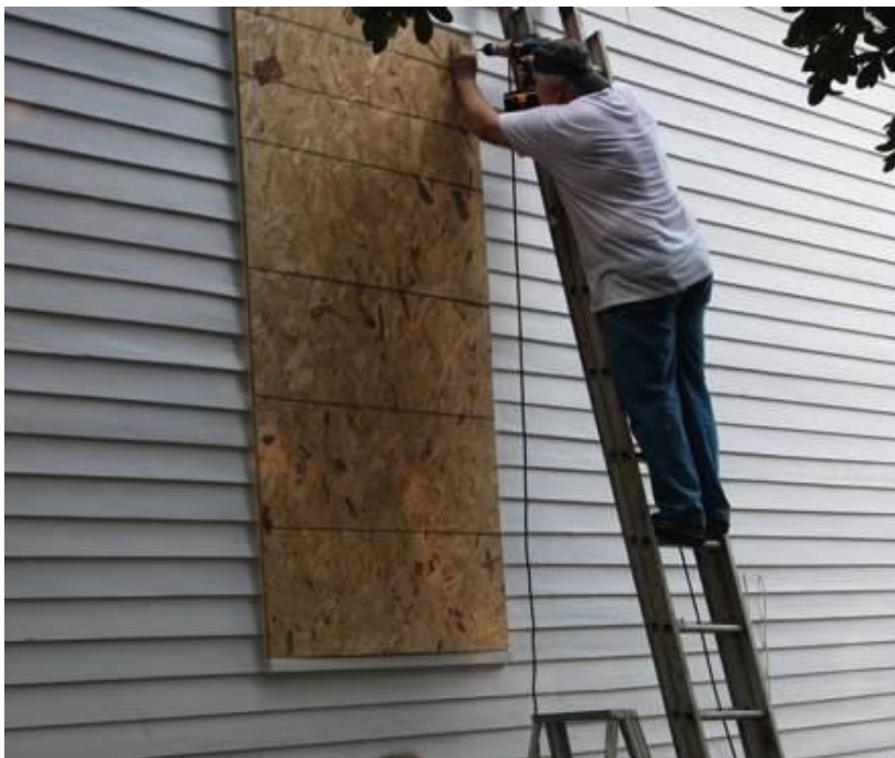
A Louisiana resident boards up his home before evacuating in preparation for Hurricane Gustav.
